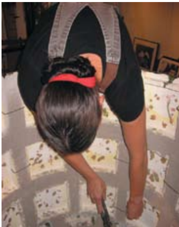
Kacheln are set first with mortar (which is 25% grog and 75% clay) and wire "staples." The flue structure is built inside, layer by layer, from the ground up.
